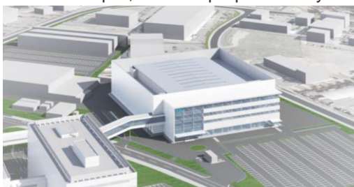
Koshi-city, Kumamoto Prefecture (Completion scheduled for summer 2025)
