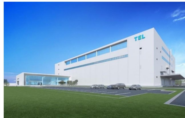
New building at the Tohoku plant
